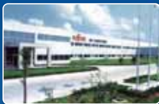
FUJITSU GENERAL (SHANGHAI) CO., LTD.
