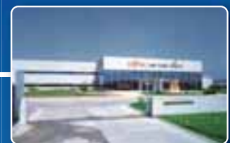
FUJITSU GENERAL (THAILAND) CO., LTD. FUJITSU GENERAL ENGINEERING (THAILAND) CO., LTD.
