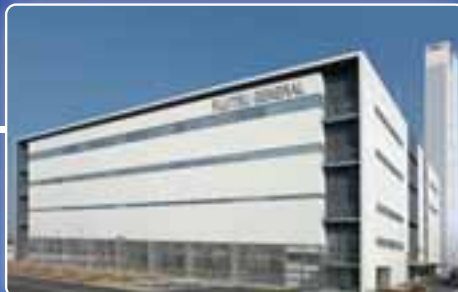
KAWASAKI R&D CENTER and 60m height difference testing tower
